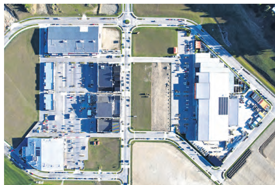
Above left: The front of the Town Centre with the new building at 89 Sir Tim Wallis Drive.
